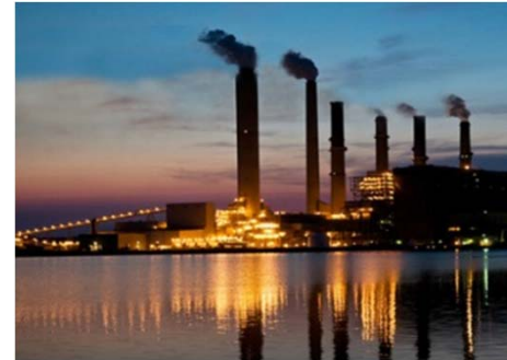
Post-Combustion Capture Retrofit
