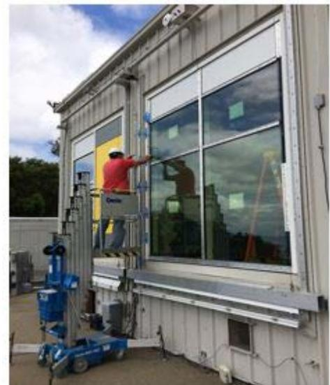
Figure 3: Installation of Sage Electrochromic Windows in the LBNL Advanced Windows Testbed
