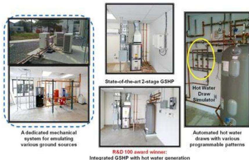
Figure 10: Major Equipment of the Flexible Research Facility for DGSHP Systems
